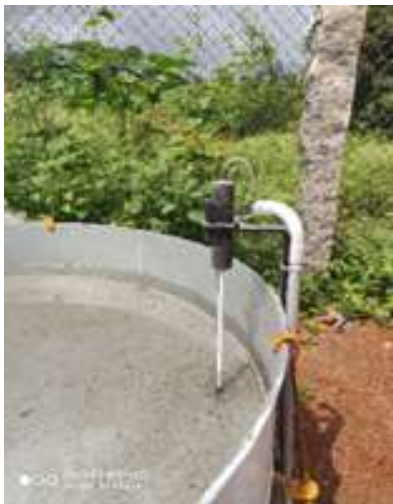
Evaporation sensor installed on a pan.
